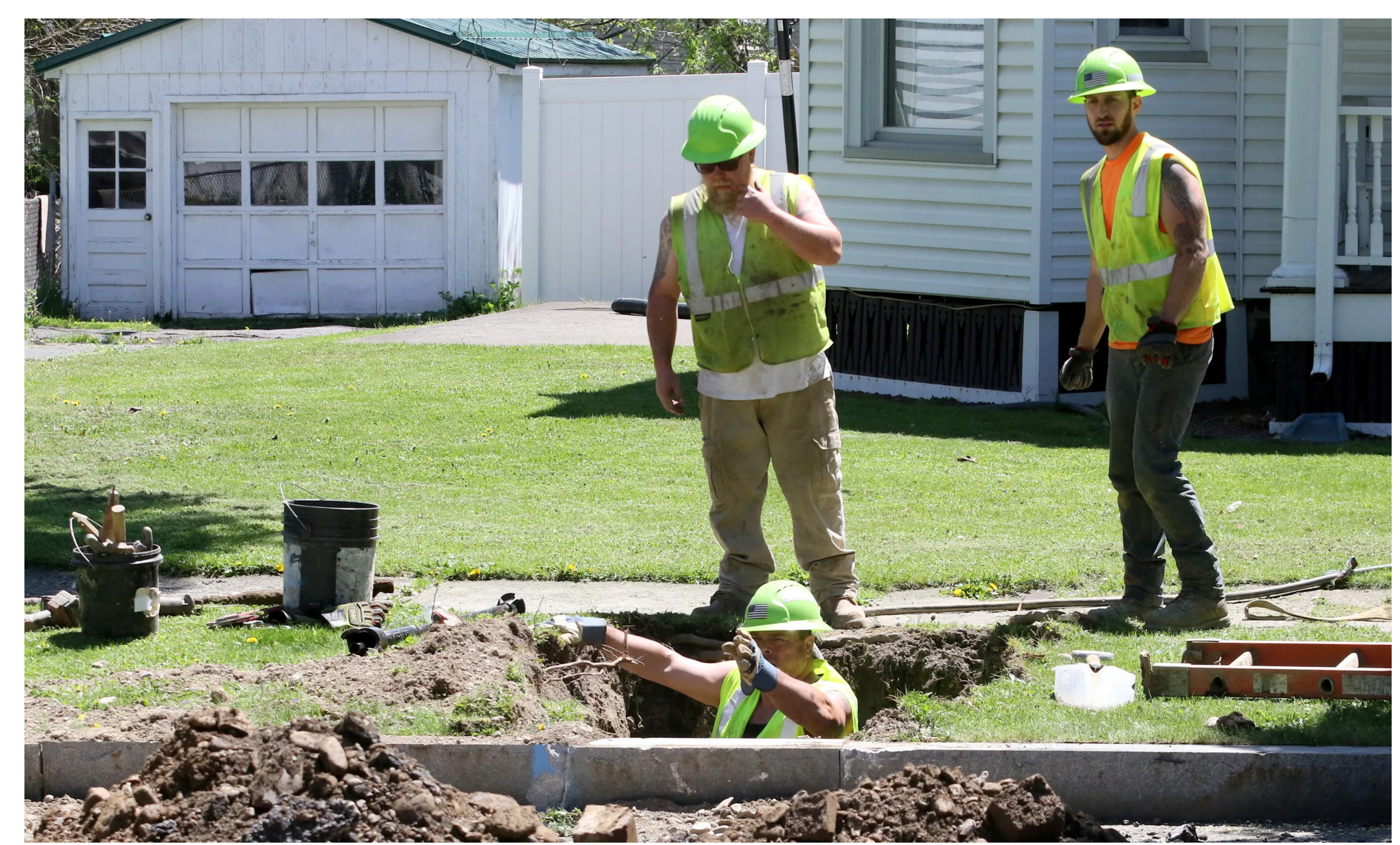
Lead pipe replacement in Elmira, courtesy of Press & Sun Bulletin, June 2022
