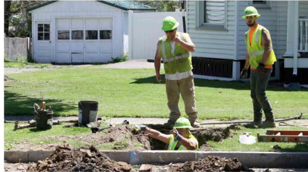
Lead pipe replacement in Elmira, courtesy of Press & Sun Bulletin, June 2022
